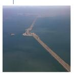
The tidal barrage makes use of a seawall constructed in 1994 for flood mitigation and agricultural purposes. Ten 25.4 MW submerged bulb turbines are driven in an unpumped flood generation scheme; power is generated on tidal inflows only, and the outflow is sluiced away. This slightly unconventional and relatively inefficient approach has been chosen to balance a complex mix of existing land use, water use, conservation, environmental and power generation considerations.
